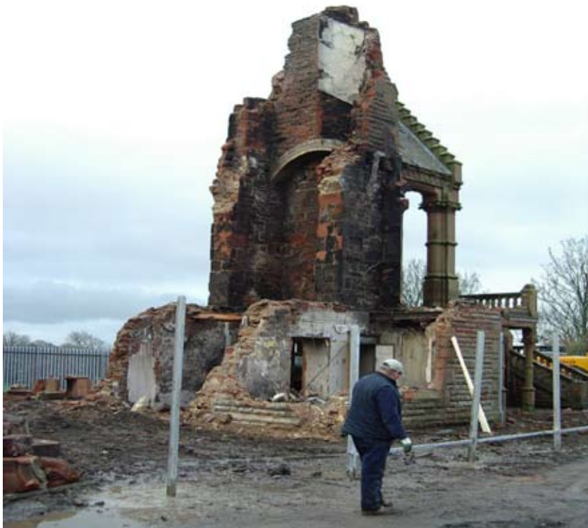
Burns Monument after November 2004 fire, Kilmarnock, Scotland (Photos: East Ayrshire Council)
