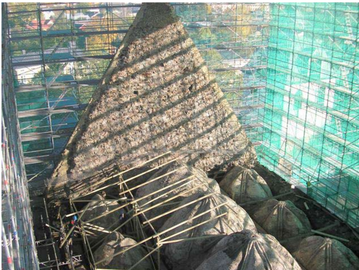
Porvoo Cathedral, Finland after October 2006 fire: (Photo: Seppo Perkurinen)
