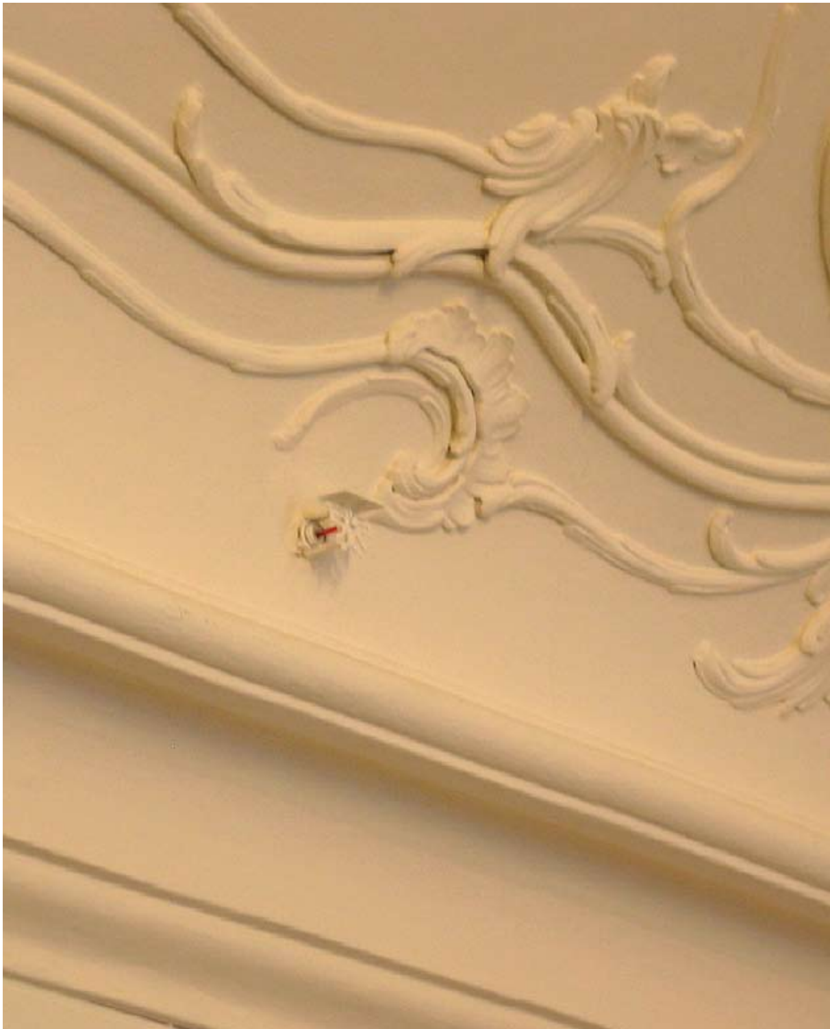
Sprinkler: (Photo: S Kidd)
